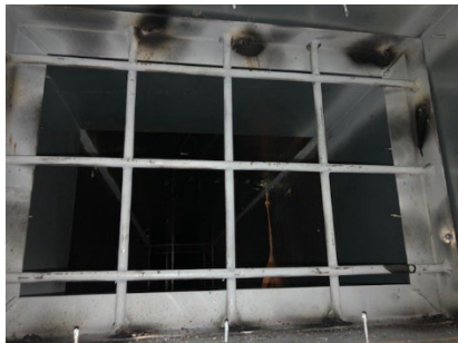
1/2 " rebar on 6" centers
